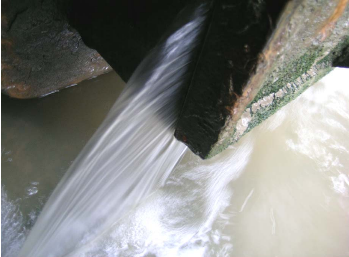
Figure 6.7: Water squirting through the gap of an almost-closed rectangular tidal flap at the mouth of a marsh drainage channel on the Thames Estuary. Even when the tide rises to the bottom of the door, this flow is too fast for elvers to overcome. As the velocity starts to fall, the gate shuts.
