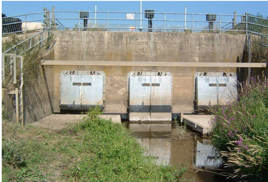
Figure 6.5: Square, top-hinged tidal flap gate
