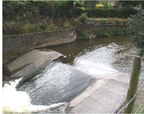
2. V Shaped broad crested weir
