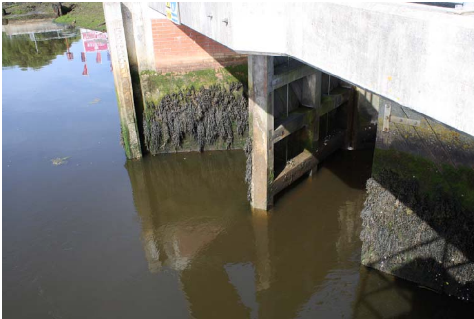
Figure 6.3: The estuary of the River Lymington in Hampshire. These tidal doors are in an open position. The tide has started to flood. The picture shows noticeable landward flow through the structure (towards the right of the picture). A few minutes later, as the landward flow increased, the doors slammed shut.
