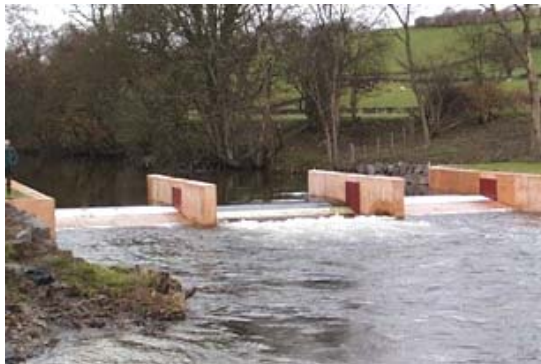
3. Compound crump. Central low section.
