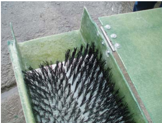
Bristle substrate (100mm width x 2) Fixed with stainless steel, self-tapping screws
