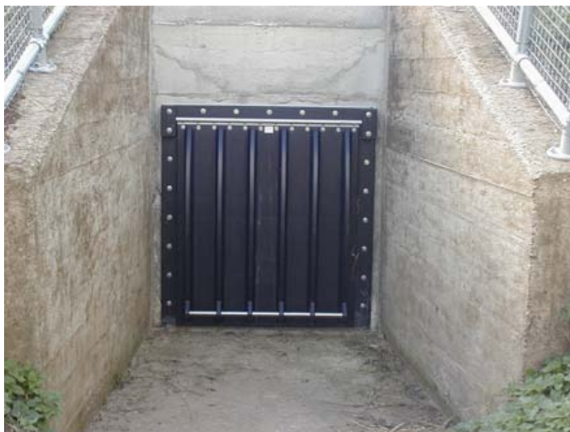
Figure 7.21: A light-weight HDPE tidal flap, manufactured by Aquatic Control Equipment (ACE) Ltd. Photograph courtesy of ACE.
