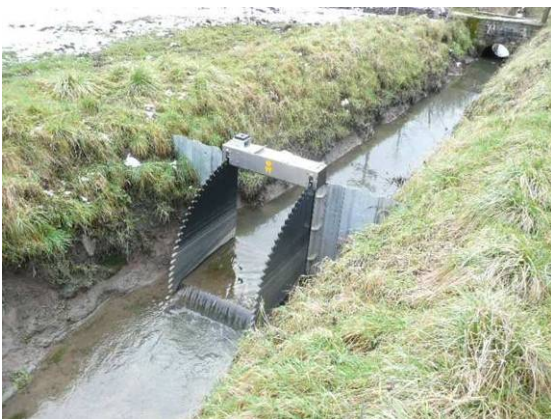
I. Pre-fabricated tilting weir
