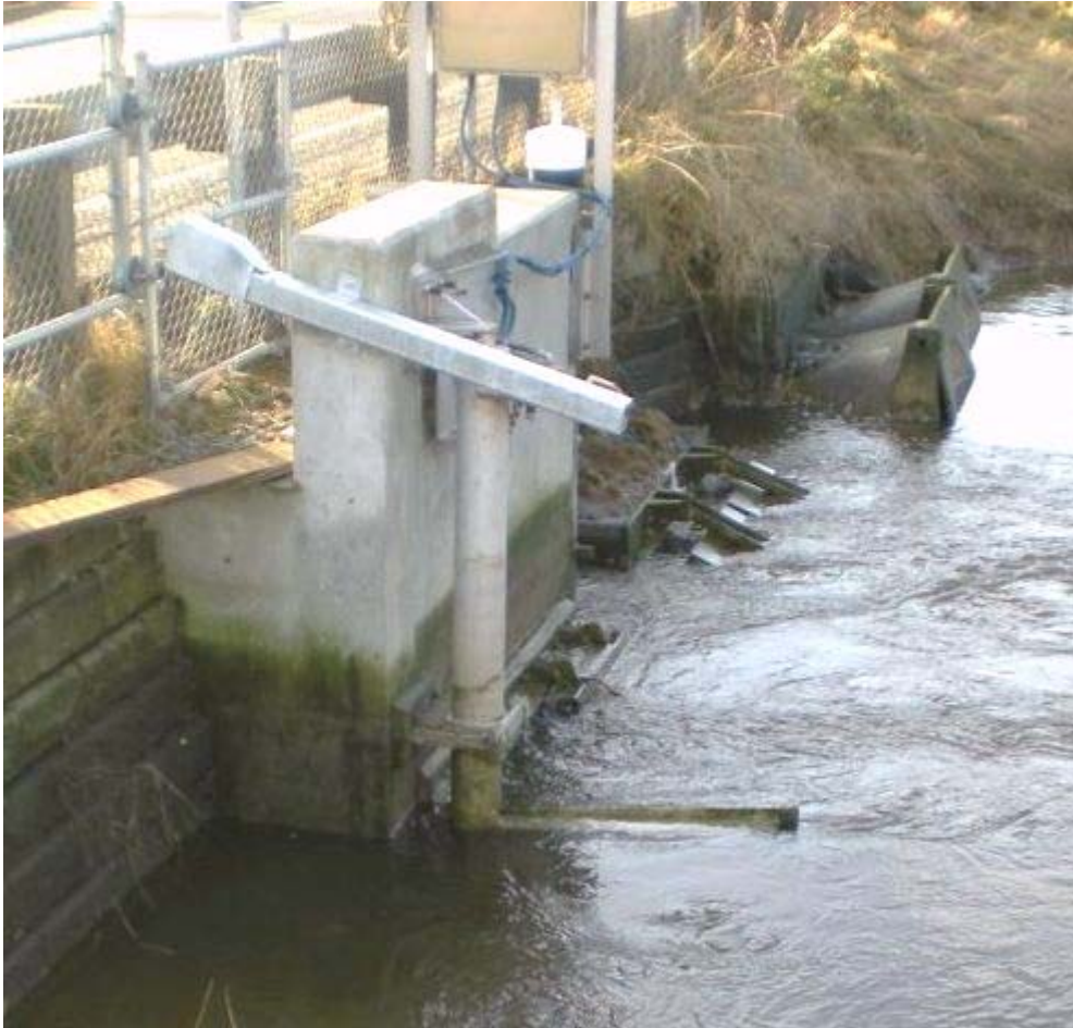
Figure 7.9: Juel Variable Backflow Flap Gate (VBFG™). The gate is fully open, on the ebb tide. Photos reproduced with permission from Juel Tide Gates of Seattle, Washington, US ( www.jueltide.com ).
