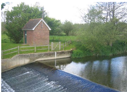
Figure 4.2 Single crump weir
