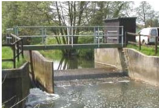
Figure 4.3 Compound Crump weir
