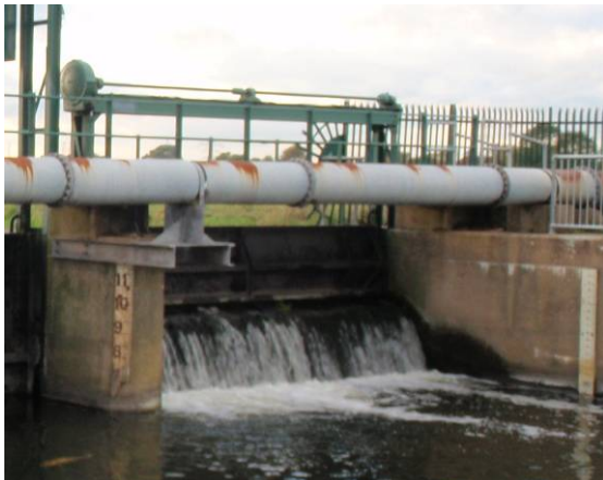
C. Small penstock sluice
