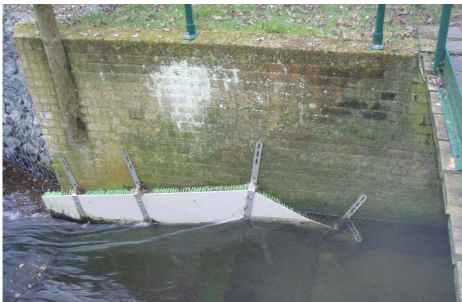
Figure 4.1: Crest section of installed pass
