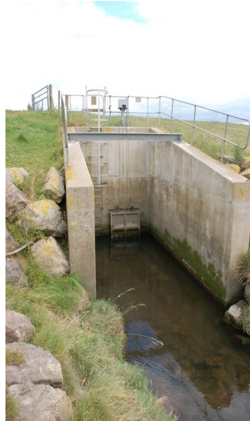
Figure 7.20: A flap gate at Warth Brook, Gloucestershire. The gate's correct invert level allows continuous opportunity for fish passage.
