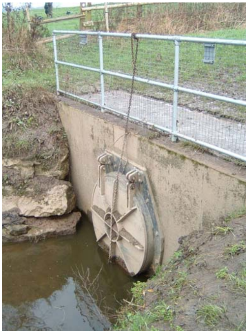
Figure 6.4: Round top hinged tidal flap gate
